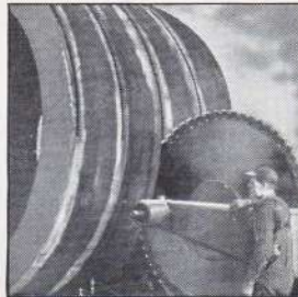
1930 Disston made world's largest metal-cutting saw, weighing 3,100 lbs., 110" in diameter.
